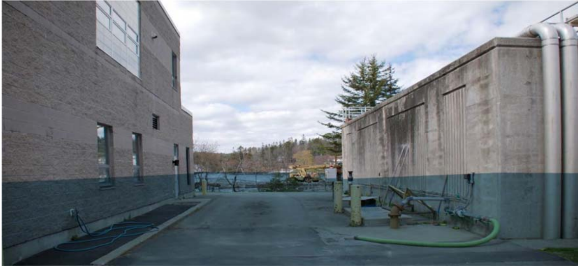
BBH WWTP Looking North Between the Process Building and SBRs – Base Flood Elevation +5 feet
